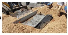
Next, we're going to set the ramp into place, making sure it sits flush on the ground. A can of spray foam comes with the kit to fill in any gaps between the ramp and the concrete border to minimize movement and prevent debris getting between the ramp and the outer edge.
