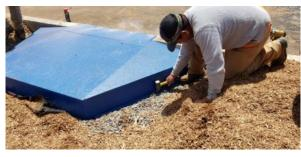
Once the threshold is mounted, anchor the base with the galvanized stakes that come with the ramp kit. There are angled brackets with various holes along the sides to drive the stakes down into the subsoil to anchor the base.
